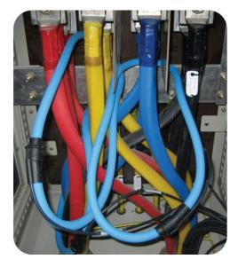
EnergiSensor Current Transformers (CTs) support our full line of revenue-grade EnergiAnalyzers and help meet all measurement and verification-based requirements. Designed as part of a simple and effective process for accurately capturing power consumption, CTs are easy to specify and install non-invasively for retrofits or new construction projects.
